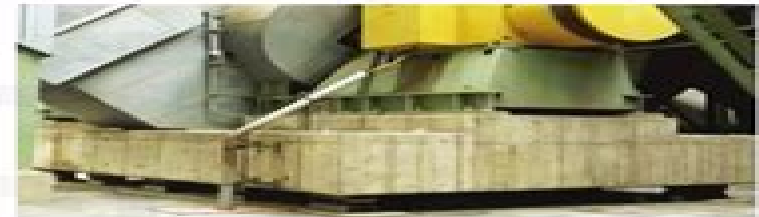
Fig. 6.3.3a—Isolator-supported fan foundation (photo courtesy of GERB Vibration Control Systems, Inc.).
